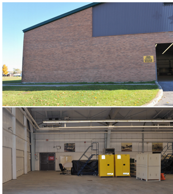
Figure 6: Photographs of the garage building.
